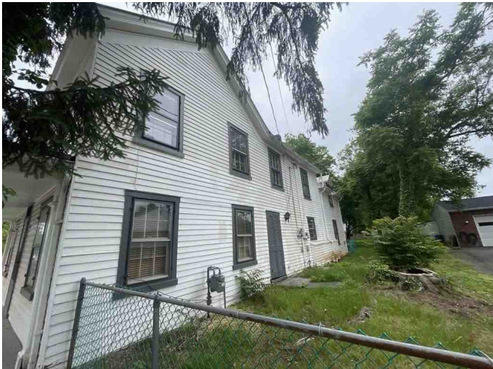
NATURAL GAS METER
