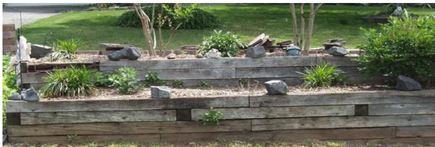
Wood Retaining Wall
