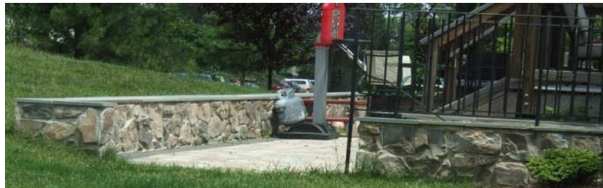
Stone Retaining Wall
