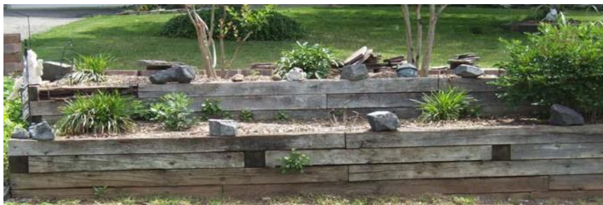
Wood Retaining Wall
