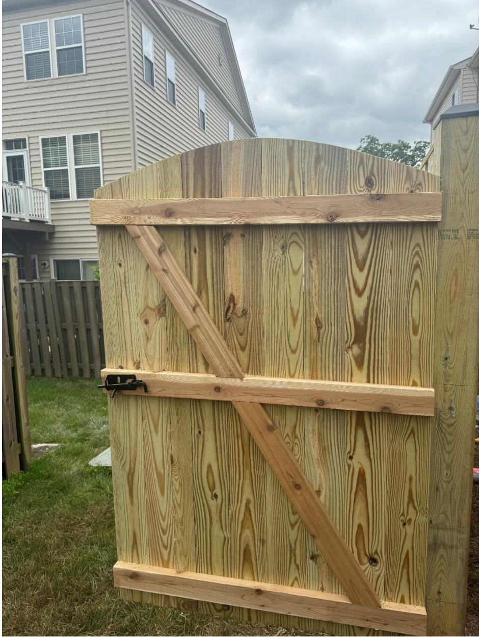
Alternate Gate with curved pickets, cedar railing, 6 x 6 post and black gate hardware
