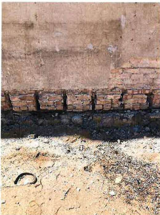
Photograph #10: Rotted Wood Plate
