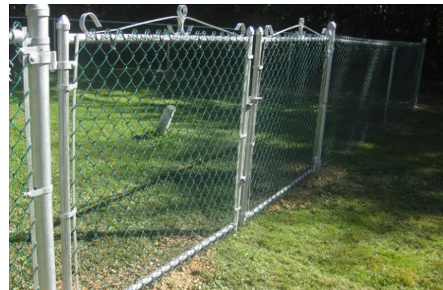
Chain link fence
