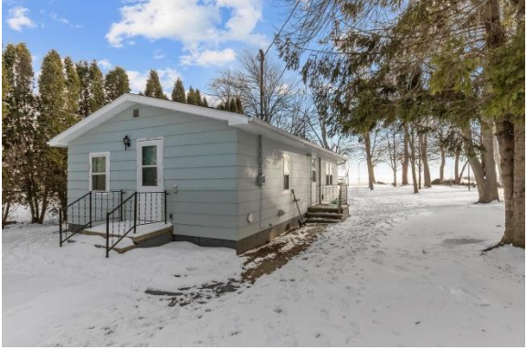
House and garage prior to renovations. Power lines between house and garage.
