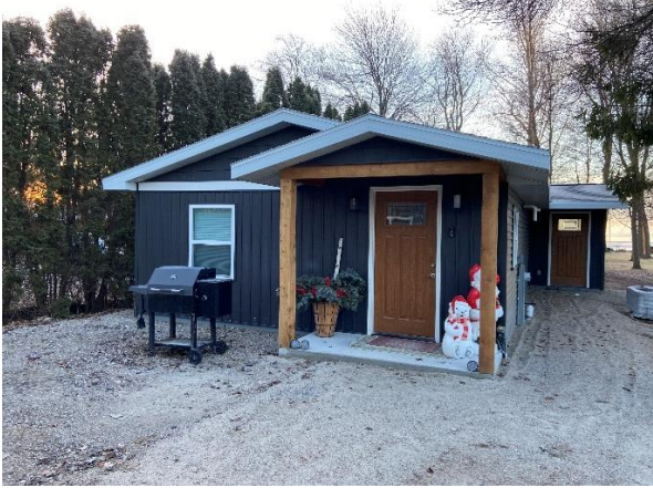
Garage after renovations. The footprint of footprint of The garage increased from 12 x 20' to 24 x 36'
