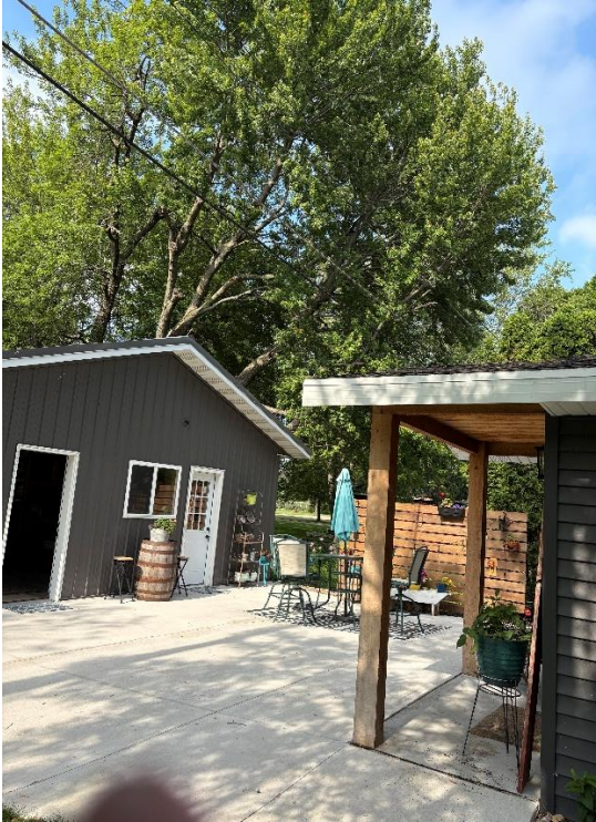
Power lines running between home and garage.
