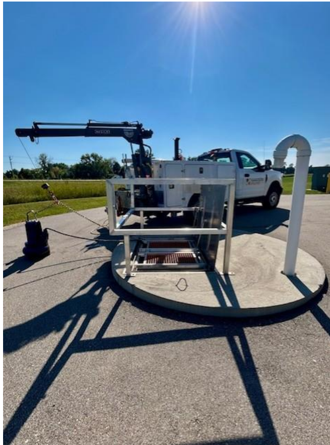
Pump removal from the Lift Station #6 Wet Well Using the Truck-Mounted Crane
