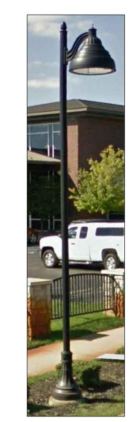
20-FT HGT. POLES AT STAGGERED APPROX. 100-FT SPACING [TO MATCH EXISTING ALONG ENTRANCE R.O.W TO NORTH]
