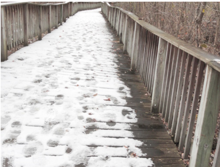
Figure 1: Sidesway displacement, towards right in photo
