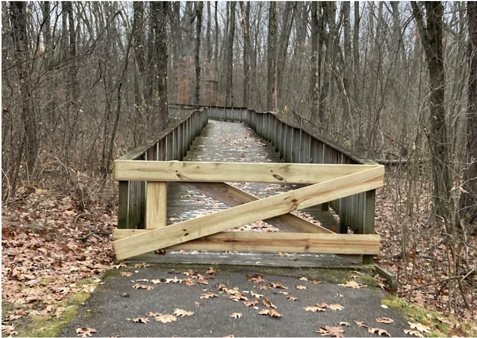
Figure 2: Beginning of boardwalk, currently closed to public access
