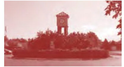
15 – Hamburg & Hall Road Historical Sign Bed
