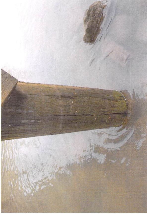
Bridge No. 0445 Br. Name Good River Date 05/17/19 Inspector McRae / Murray Frame 22 P3 DS pile vertical splits File P5170625.JPG
