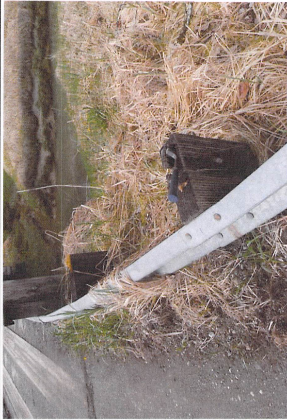
Bridge No. 0445 Br. Name Good River Date 05/17/19 Inspector McRae / Murray Frame 16 NE US approach railing post, typ. File P5170622.JPG
