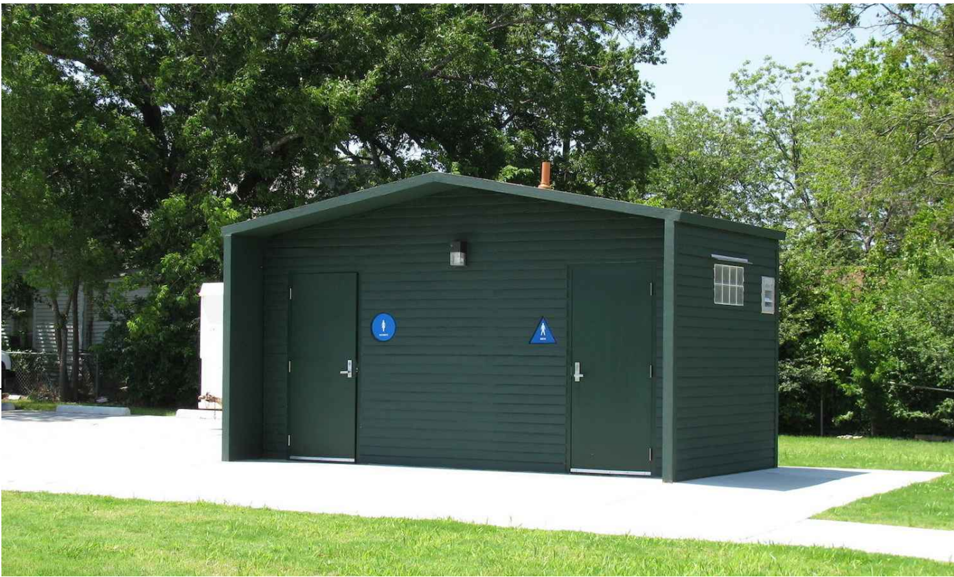
PRE-FABRICATED PUBLIC TOILET FACILITY WITH DRINKING FOUNTAIN + BOTTLE FILL, EQUIPMENT STORAGE SHED + HOSE BIBB CONNECTION. [CONCEPT IMAGE]
