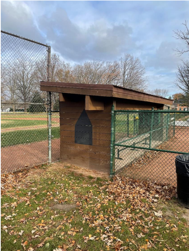
New Dugout and fencing replaces brown wooden existing structures.
