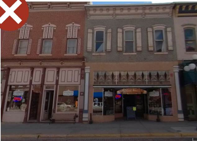
No covered walkway or awning incorporated in the adjacent public right-of-way.
