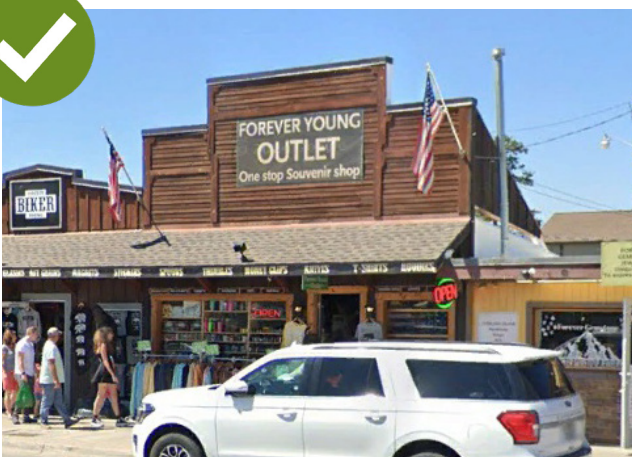
Flat roofs feature a false parapet.
