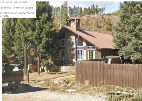
EXISTING BUILDING PHOTO
