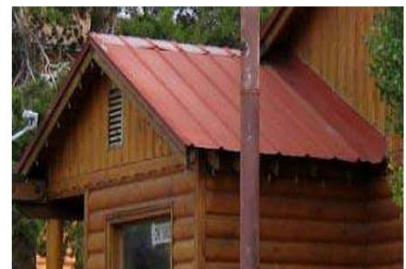
STANDING SEAM ROOF TO MATCH EXISTING
