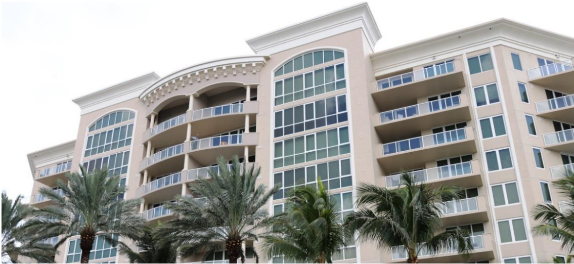
Different shapes and building forms create a diverse top articulation. 18
