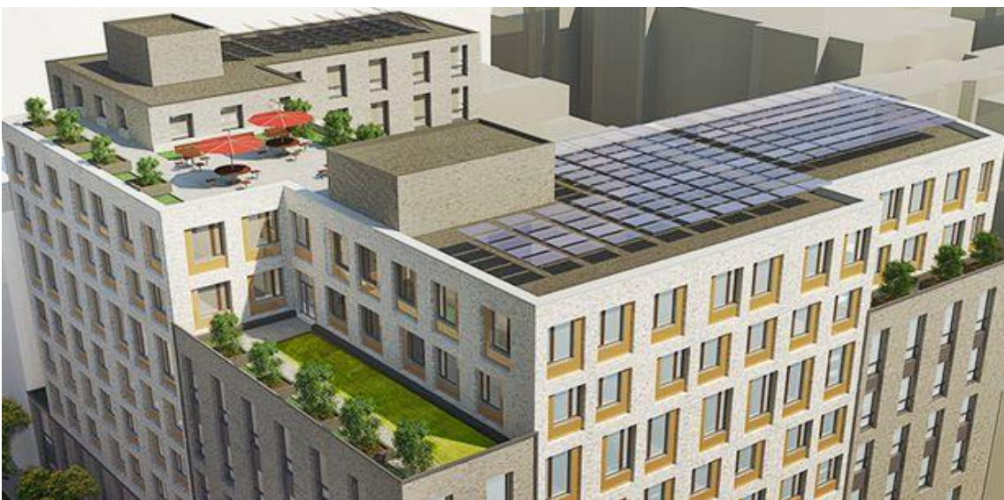
The roof design creates comfortable and enjoyable recreational spaces, providing amenities and pleasing views to the surrounding built and natural environment. 19
