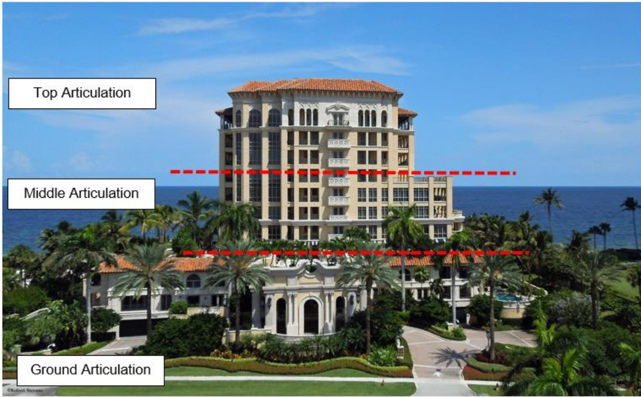
Various building articulations provide visual diversity a sense of human scale, and minimizes the massiveness of buildings. 16
