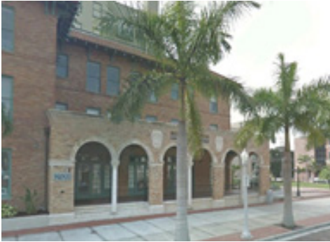
Figure 4.4: Building with gallery
