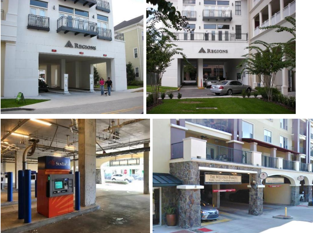
Figure XIV - 44. Interior Drive-Through Facilities
