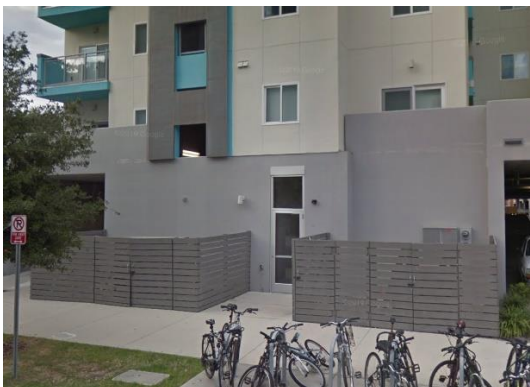
Allowed (utilities screened by fence)
