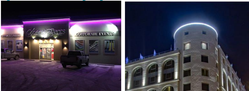
ABOVE: LED rope lights outlining the building cornice (permitted) BELOW: String lights outlining the cornice
