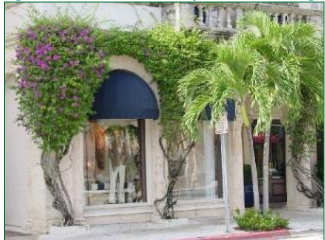
Figure XIV - 56. Planters Adjacent to Buildings
