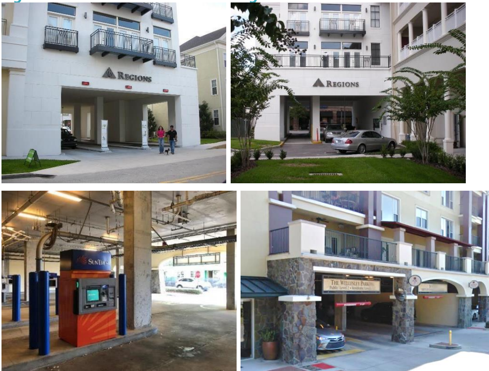
Figure XIV - 47. Interior Drive-Through Facilities
