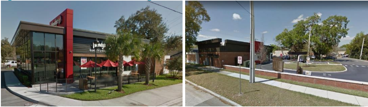
Examples of appropriate design for drive-through facilities (building up to the street; drive-through window in the rear)
