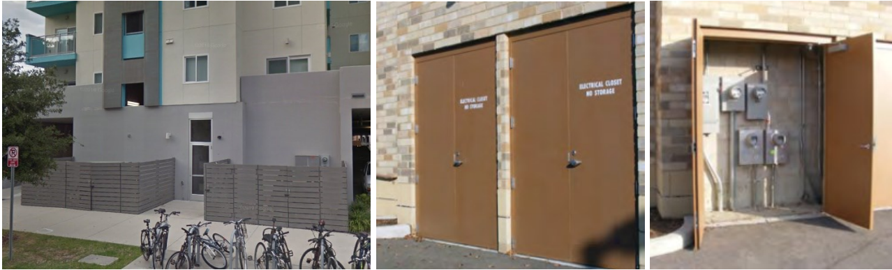
Allowed (utilities screened by fence)
