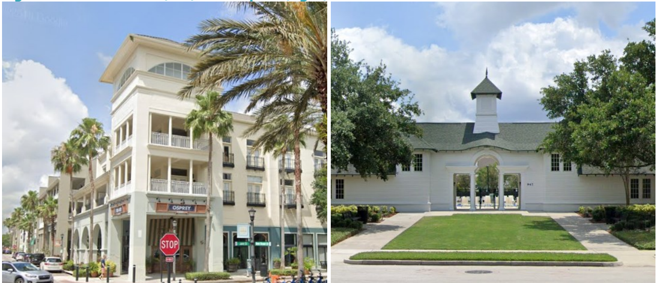
Figure XIV - 16. Tower (left) and Cupola (right)
