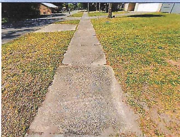
Figure 11. Sidewalk Uplift & Spalling, Martin Luther King Jr. Blvd
