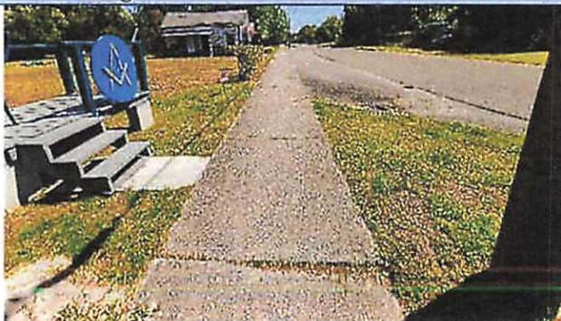
Figure 11. Sidewalk Uplift & Spalling, Martin Luther King Jr. Blvd
