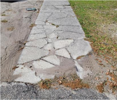
Figure I-2. Sidewalk Cracking & Loss, Martin Luther King Jr. Blvd
