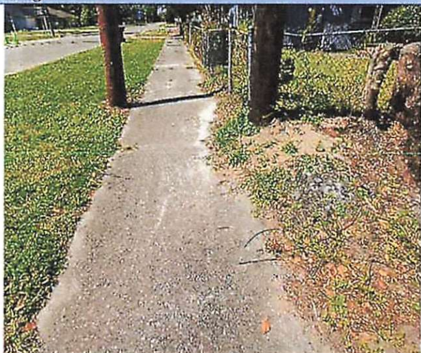
Figure 9. Sidewalk Spalling, Martin Luther King Jr. Blvd
