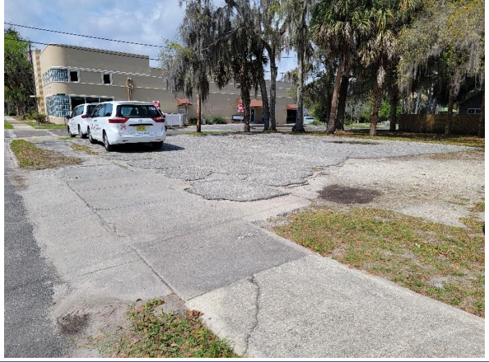
Figure 44. Vacant Lot, East of 604 Walnut St
