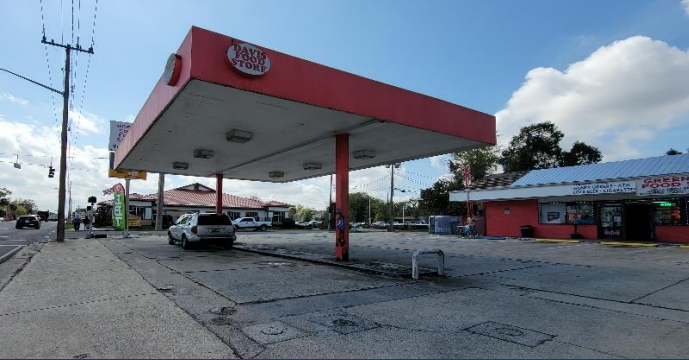
Figure 21. Unsafe, Low hanging power lines, concrete drive in disrepair, south of 25 N Orange Av
