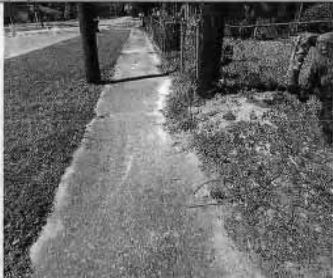
Figure 9. Sidewalk Spalling, Martin Luther King Jr. Blvd
