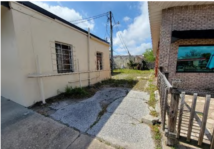
Figure I-21. Unsafe, Low hanging power lines, concrete drive in disrepair, south of 25 N Orange Ave
