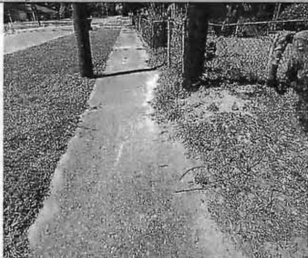
Figure 9. Sidewalk Spalling, Martin Luther King Jr. Blvd
