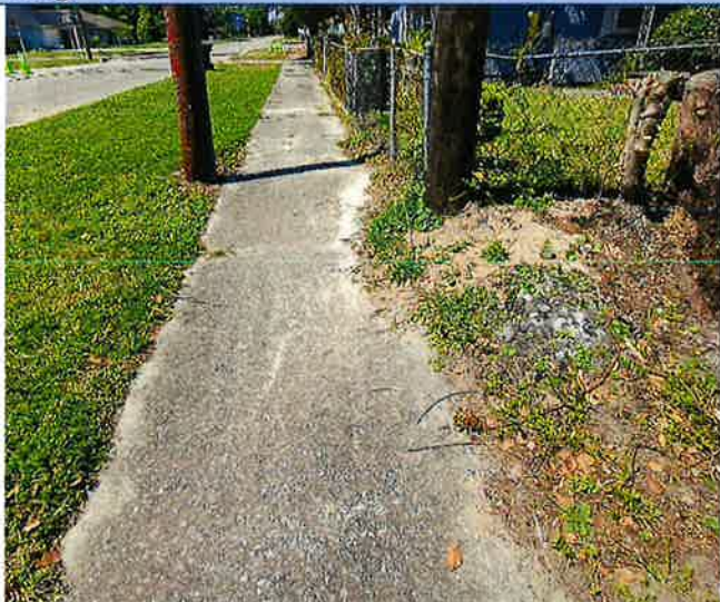
Figure 9. Sidewalk Spalling, Martin Luther King Jr. Blvd
