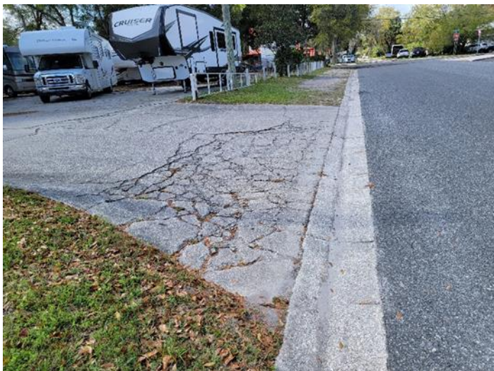
Figure I-31. Deteriorating Drive, 327 N Orange Ave
