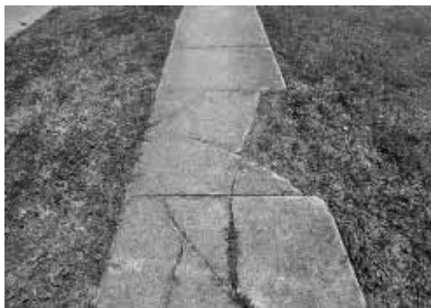
Figure I-3. Deteriorating accessibility feature, Corner of Orange Ave & Center St
