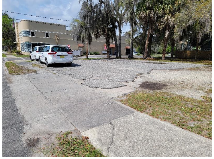
Figure 44. Vacant Lot, East of 604 Walnut St
