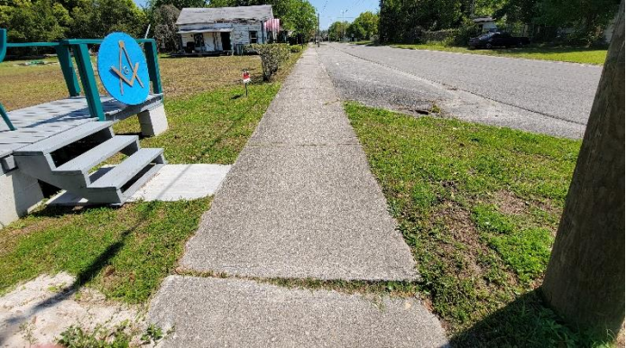
Figure 11. Sidewalk Uplift & Spalling, Martin Luther King Jr. Blvd
