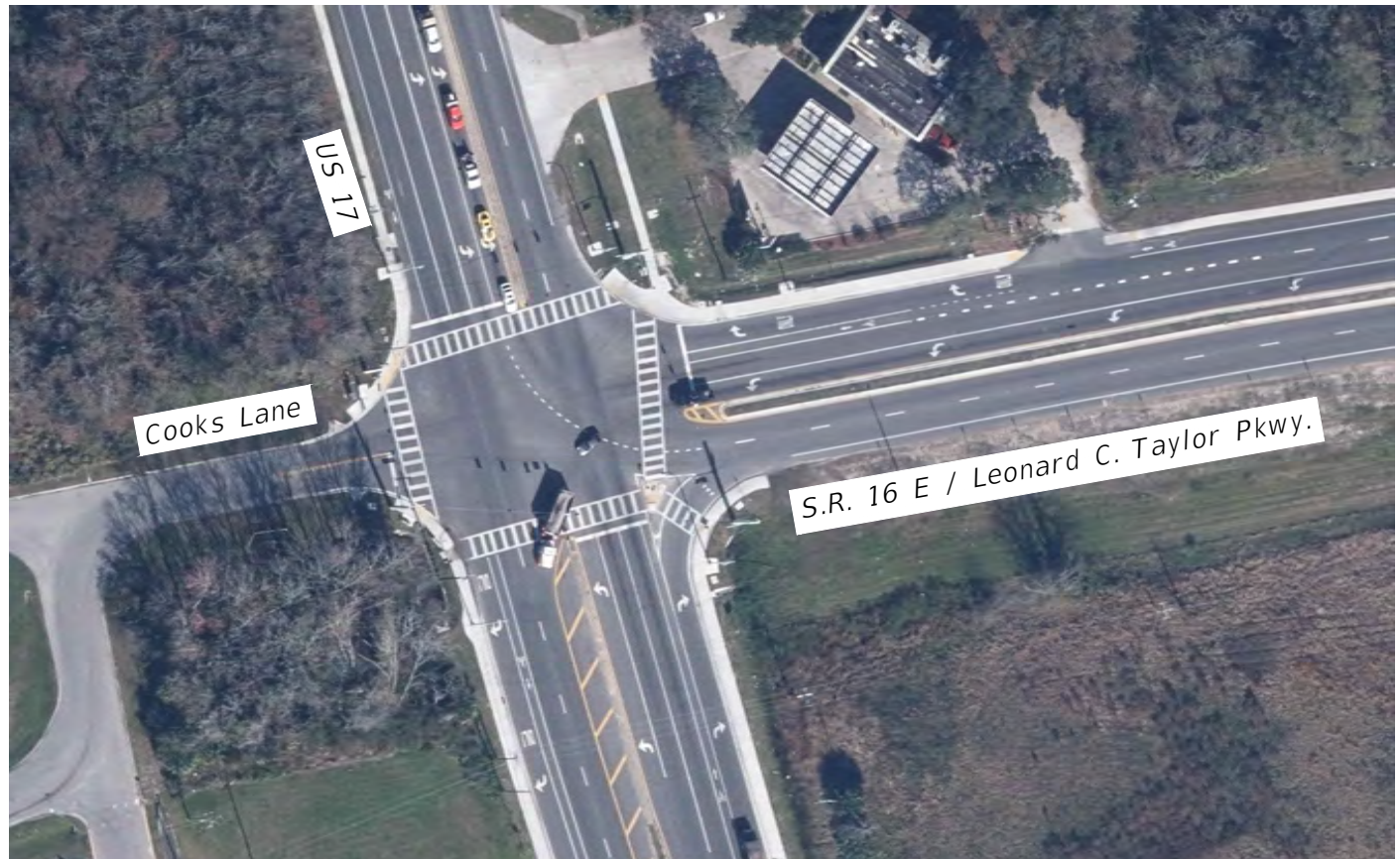
US 17 at Cooks Lane and S.R. 16 E. / Leonard C. Taylor Pkwy.
