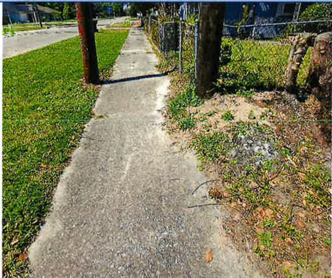
Figure 9. Sidewalk Spalling, Martin Luther King Jr. Blvd
