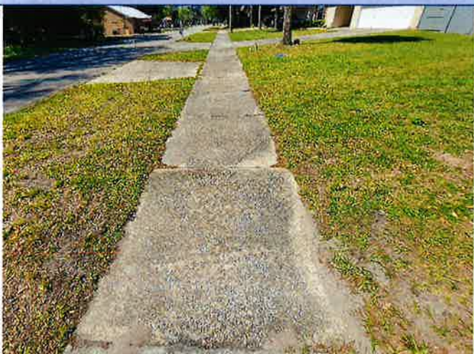
Figure 11. Sidewalk Uplift & Spalling, Martin Luther King Jr. Blvd
