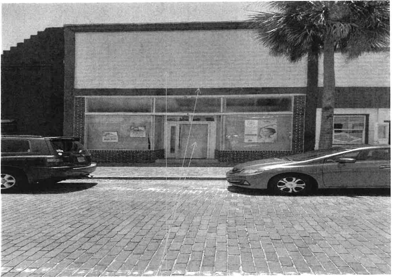
Pressure wash, prep and apply two applications of finish on walls, trim and door.
