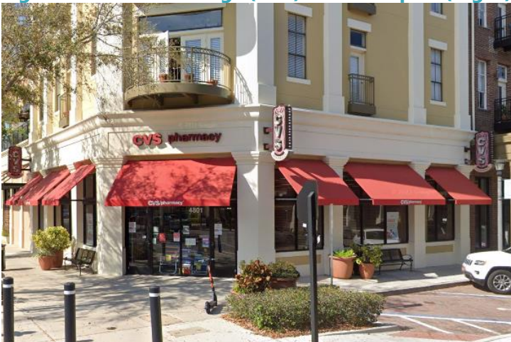
Figure VIII - 23. Awnings (Left) and Canopies (Right)
