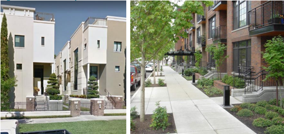
L: Combination of exterior and interior facing doors; R: Exterior facing doors
