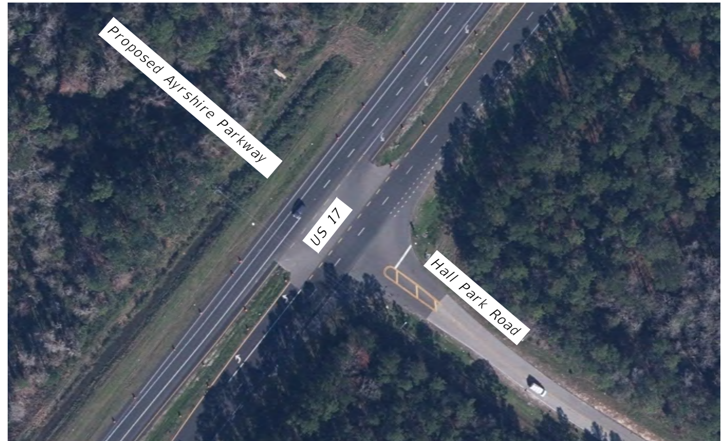
US 17 at Hall Park Road
