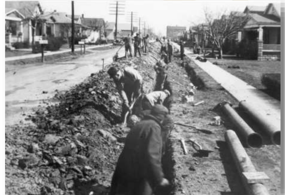
1936 photo of workers installing water pipes in an Indiana community
