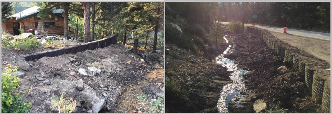
Figure 11: Structure & Road Overtopping Protection at Dry Creek. The area will be stabilized with native vegetation Fall 2021.
