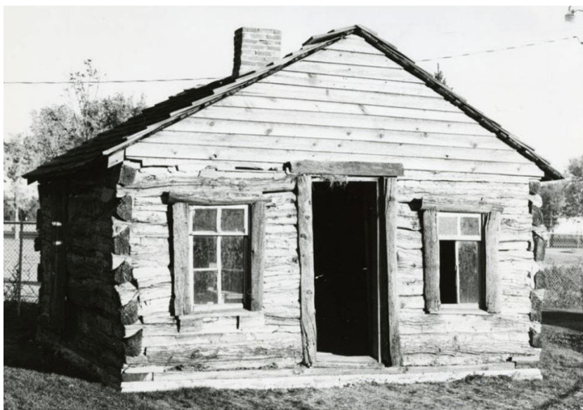
Figure 65. Original Weld County Courthouse constructed from hewn cottonwood logs with dovetail notching. This building was constructed around 1860 and relocated from its original site near Fort Vasquez in Platteville to Greeley's Centennial Village where it remains on display. AI-0464, City of Greeley Museums, Weld County Images Collection. 1979.
