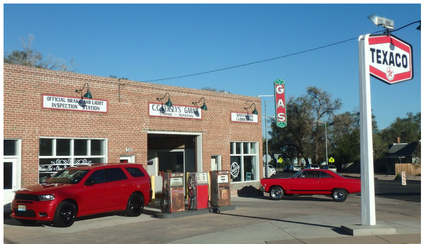
Figure 20. C.C. Kersey's Garage, 531 8th Street. This building shows the small-scale development prevalent throughout the Sunrise neighborhood which includes residential, commercial, and light industrial facilities.
