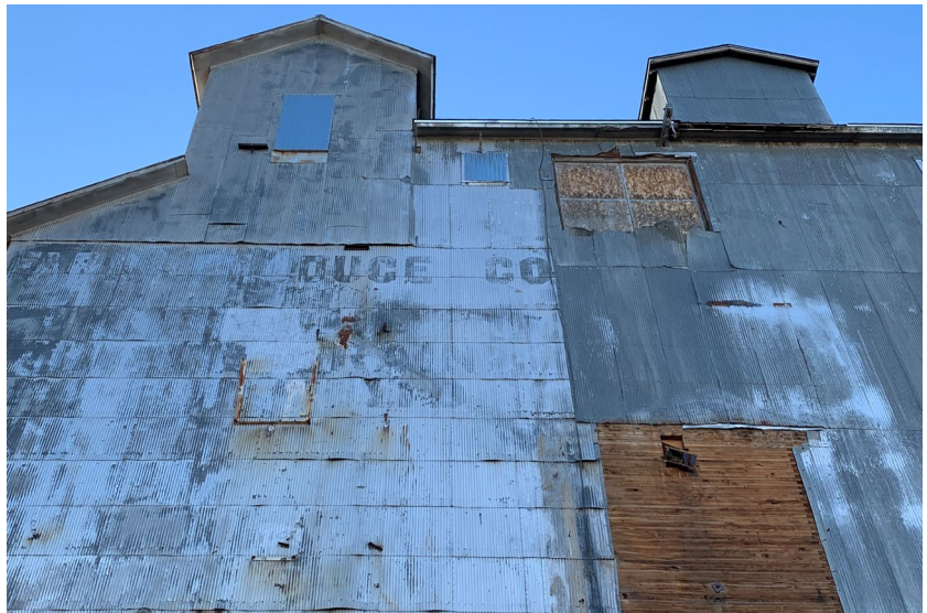
Figure 68. D&D Bean Company, 601 10th Street. An example of stacked lumber construction is visible on this elevator where the removal of exterior features has left the internal structure exposed beneath the corrugated metal skin.
