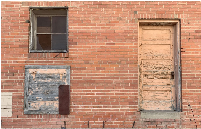
Figure 69. 701 7th Street. Detail of north elevation showing utilitarian use of brick masonry in an industrial setting.
