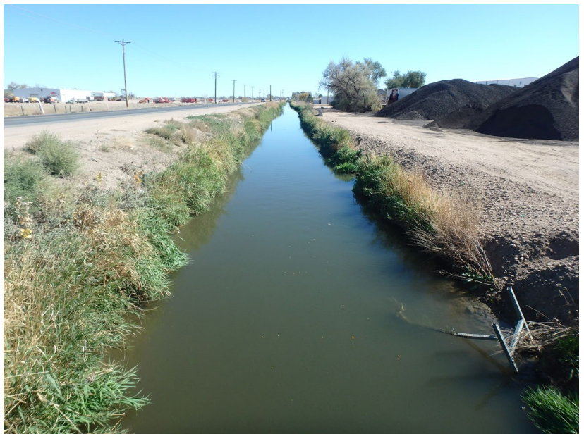
Figure 58. Portion of the Ogilvy Ditch (5WL.2944) along E. 8th Street, looking east. This ditch was originally constructed in 1881. Portions of it have been determined field eligible for the NRHP.
