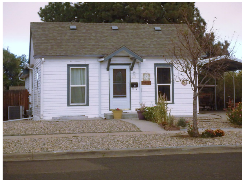
Figure 81. 419 12th Street. This residence is an example of a Hall-and-Parlor building type with its side-gable entrance and single room depth. An addition has been constructed off the rear of building to provide additional living space.
