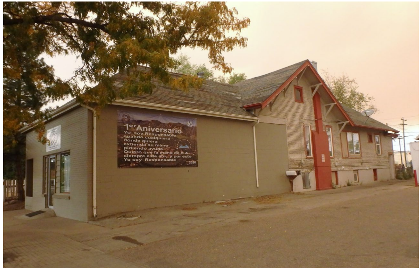
Figure 80. 705 13th Street. Here, a one-and-a-half story craftsman bungalow has been added onto with a masonry one-part commercial block which occupies its original inset porch and front yard.
