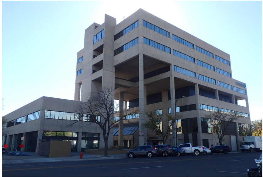
Figure 92. Greeley National Bank Building, 822 7th Street. Constructed in 1974, this is an example of a Brutalist style High Rise in Greeley’s downtown core.
