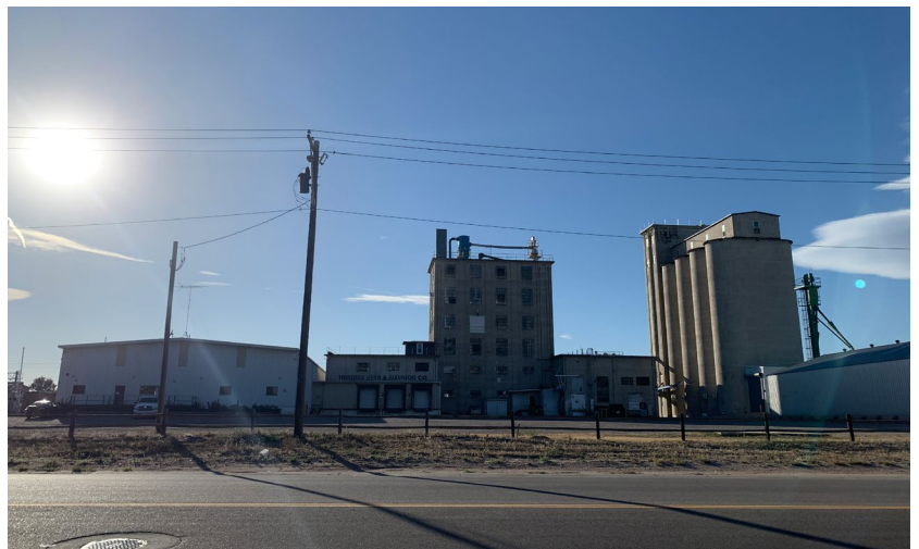
Figure 54. Trinidad Bean & Elevator Company, 615 5th Street. This collection of buildings may also form part of a cultural landscape which showcases the manner in which agricultural products were stored and transferred between rail and road vehicles.
