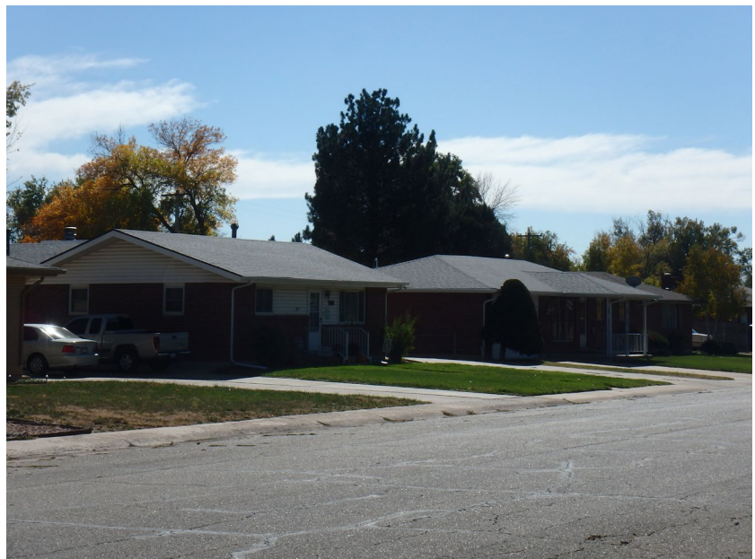
Figure 8. 2618-2622 16th Avenue. View looking southeast showing examples of archetypal American ranch houses which exist in near original condition in the Hillside neighborhood.
