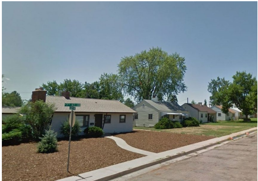
Figure 18. 2402-2414 W. 7th Street. View showing the Minimal Traditional style residences that define the architecture of the Houston Heights subdivision.
