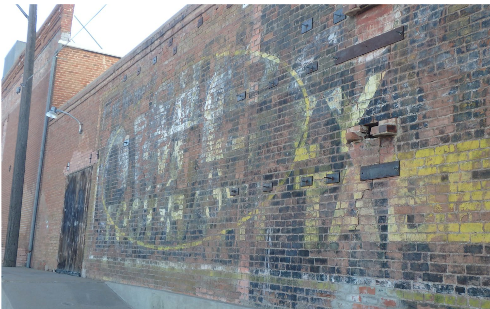
Figure 30. Hand-painted wall signs (ghost signs) on the east elevation of the Bean Plant Studio, 701 7th Street.
