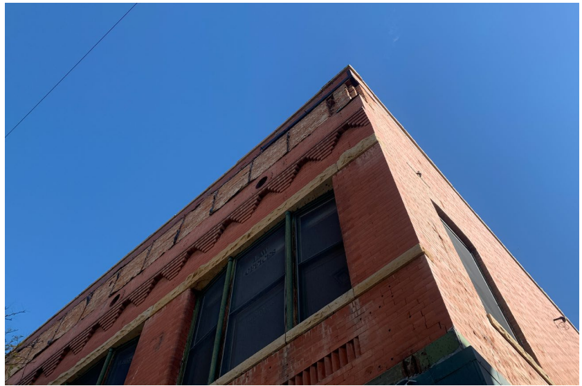
Figure 72. Coronado Building, 900-920 9th Avenue (5WL.2284). Detail of stone belt courses forming sills and lintels of upper story windows.
