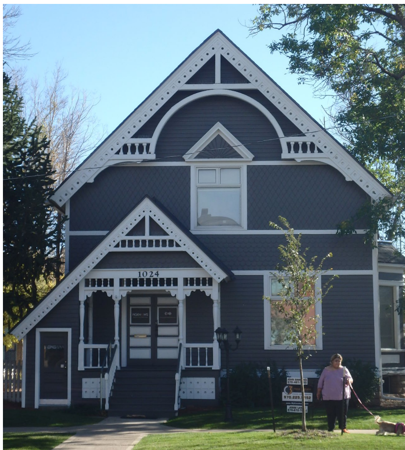
Figure 98. Boomer House, 1024 8th Street (5WL.771). Constructed in 1895, the Boomer House shows the asymmetrical composition and multi-textured wall surfaces that characterize the Queen Anne style. This building was evaluated for NRHP eligibility in 1982 but no formal determination was made by the Colorado SHPO.
