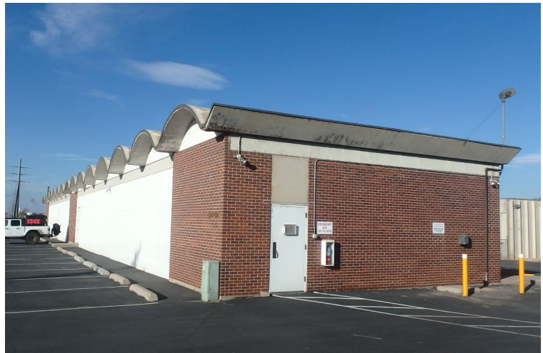
Figure 48. Hensel Phelps Construction Co., Building 2, 420 6th Avenue. This storage warehouse with a remarkable undulated thin-shell concrete roof was constructed in 1961 according to data from the Weld County Property Portal.
