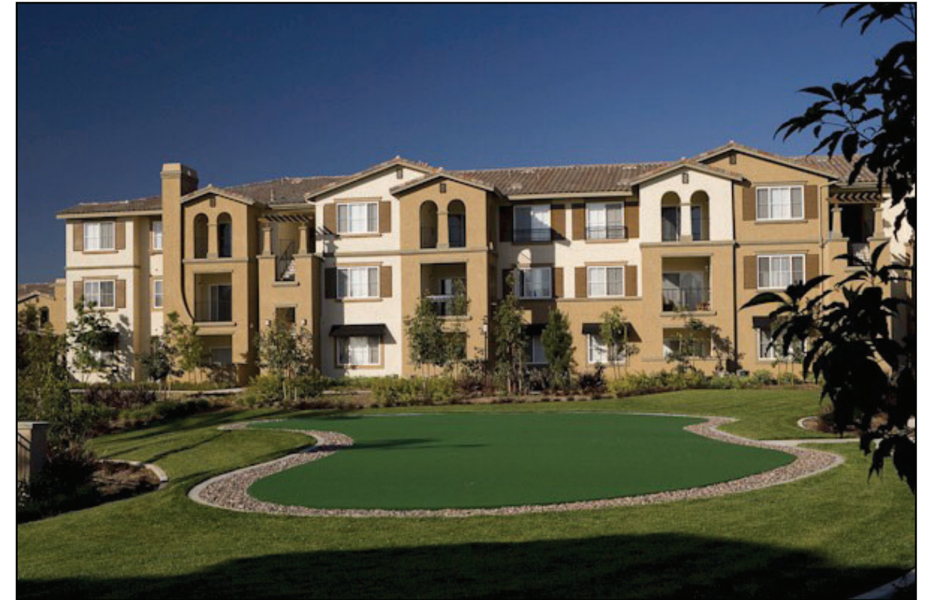
On larger multi-family buildings, architectural elements such as: variation in building elevation plane, incorporation of high profile roofing materials, real or simulated chimneys and decorative shutters shall be required.
