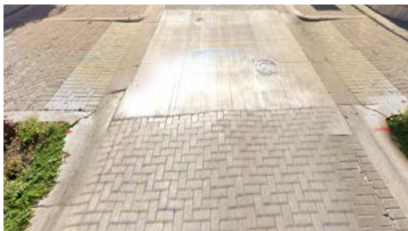
Image of existing unit pavers and colored concrete area on 8th Street needing repair and maintenance
