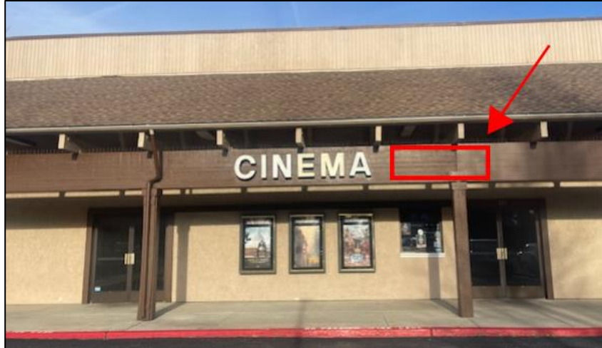
Proposed Sign Location at Building Frontage
