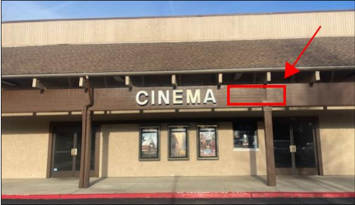
Proposed Sign Location at Building Frontage
