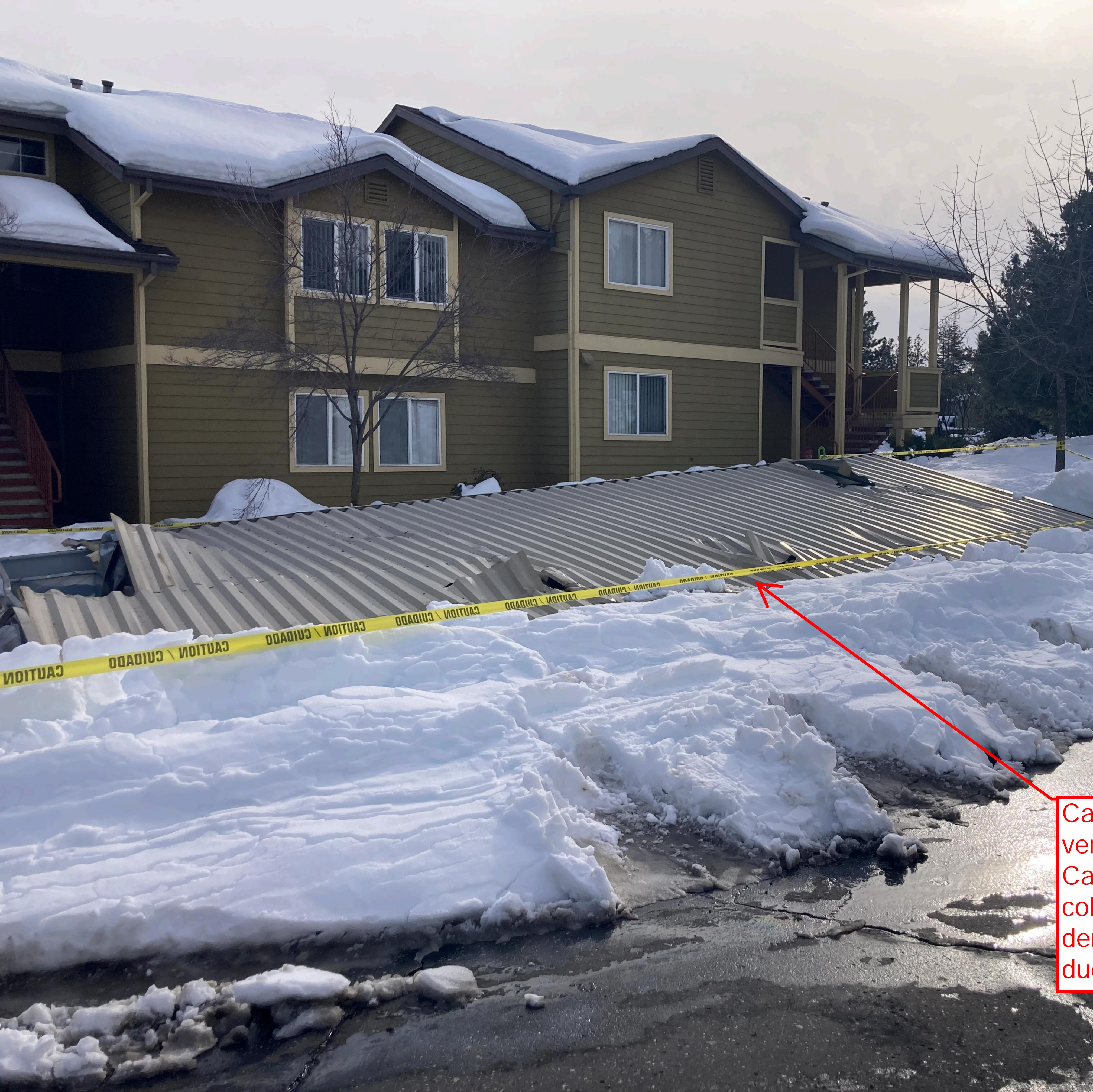
Carport was partially collapsed and was demolished immediately due to tenant safety.
