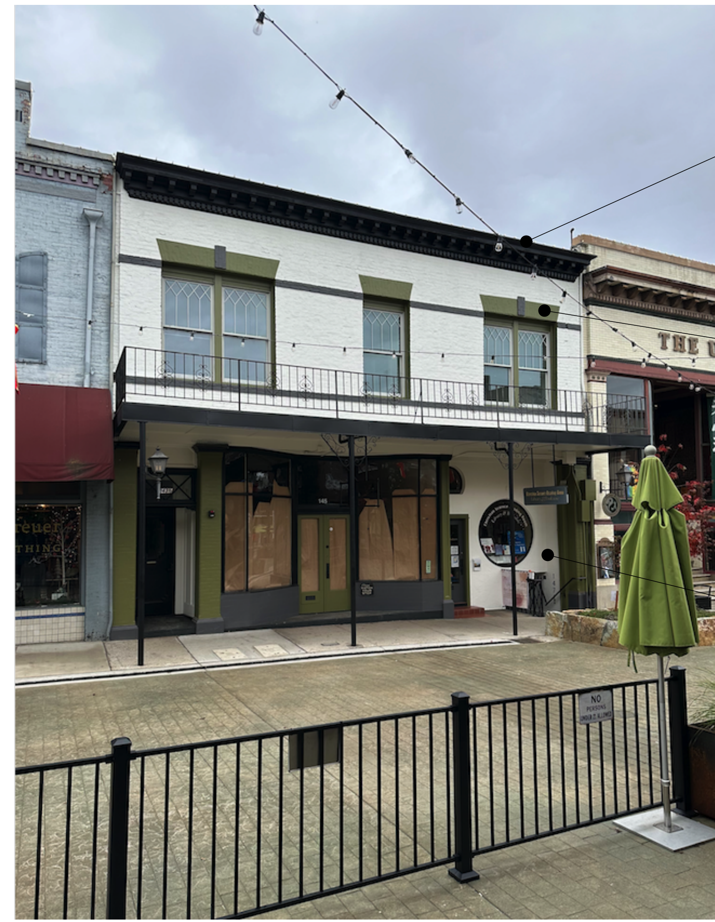
145 MILL STREET VIEW
