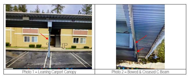
Based on provided information, our office believes significant snow loading damaged the carport structures inducing deformed and buckled structural light-gage framing members. Once light-gage members experience deformation (i.e., flange and web crippling) their structural integrity is greatly compromised, and they should be replaced. In our opinion, snow loading damaged the carport structures located at 265 Sutton Way, which now require replacement.
