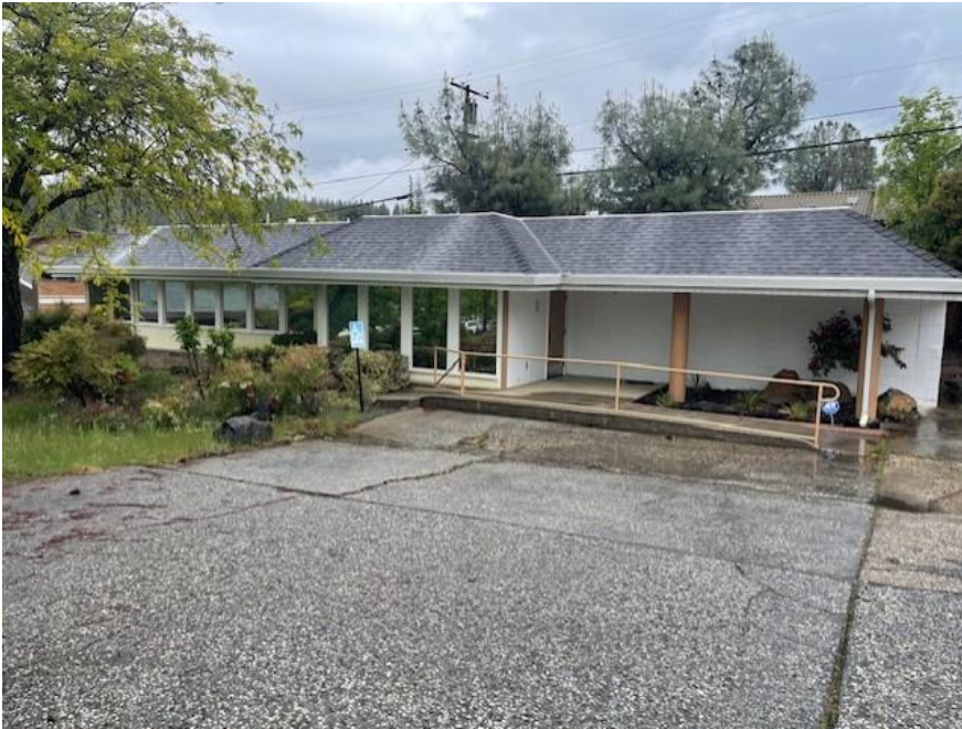
Image 1 – Front of Existing Building and Parking Lot
