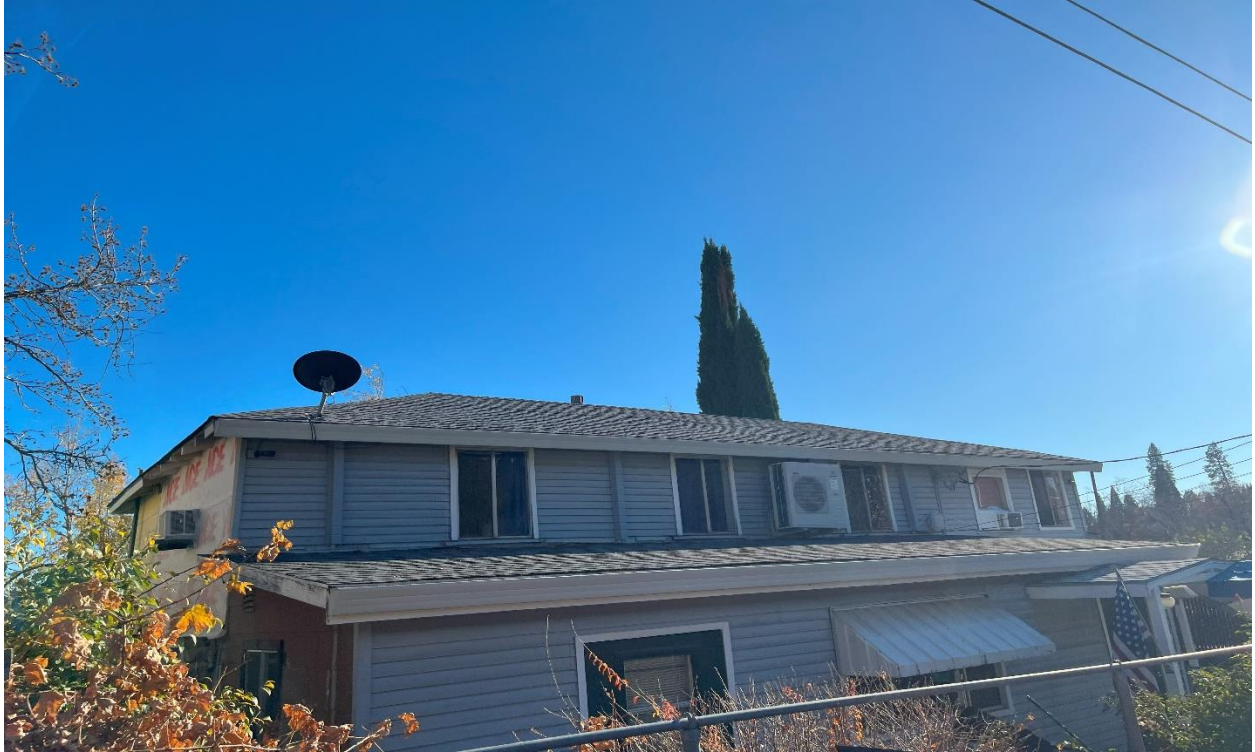
Photo 9: Existing structure within the subject parcel from along Glenwood Avenue. Only the tall non-native tree in photo and the blue oak tree encroach within the parcel.
