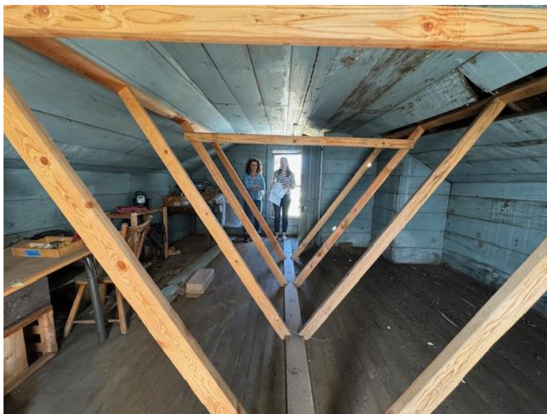
Photograph 10: View of the attic looking north.
