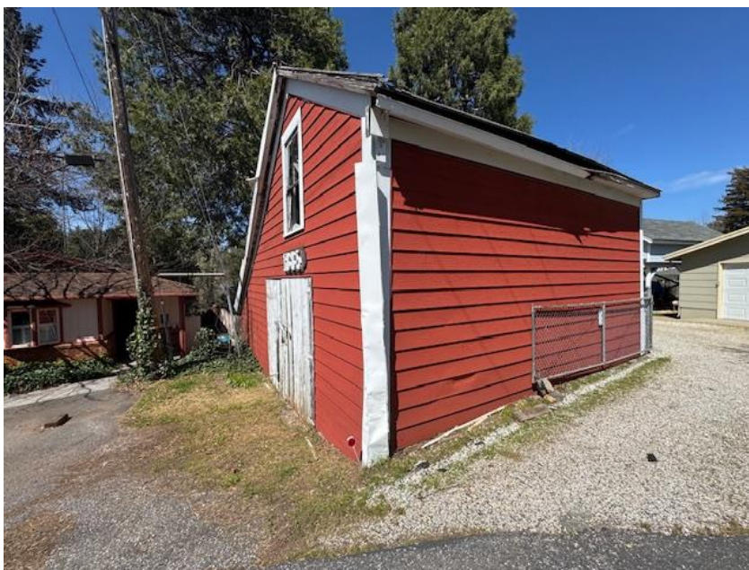
Photograph 2: View looking northwest at the southeast elevation of the barn. Note that the siding on these two elevations is aluminum clapboards.
