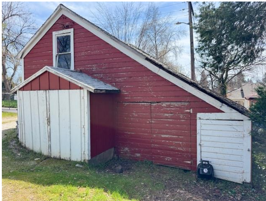
Photograph 4: View looking southeast at the north elevation of the barn. Note the shiplap siding has been cut and repurposed for the two swinging doors with a new door on the right.
