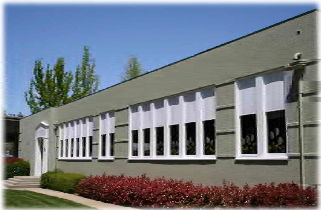
Use of a repeating ribbon type window in a Grass Valley school building.
