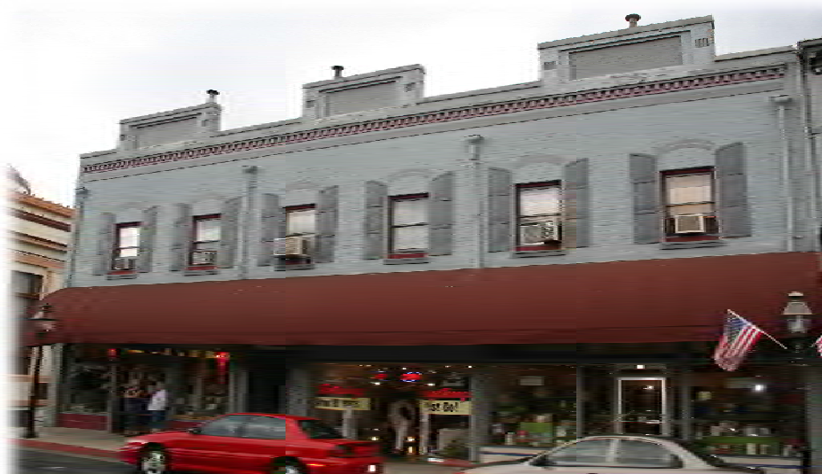
Note the second-story double-hung wood windows and arched brick lintels above each window along with flanking shutters. The only distraction is the addition of exterior mounted air conditioning units.
