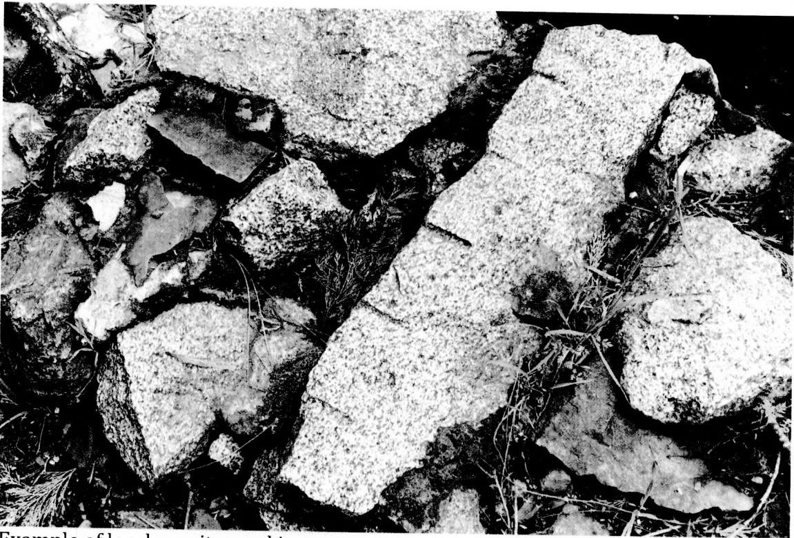
Example of local granite used in construction of the abutments.
