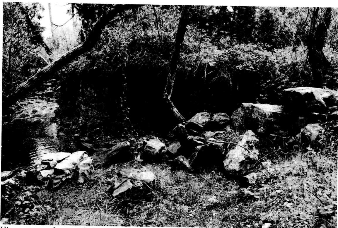
View across the trestle location from the western edge of the creek. Both abutments were designed to direct the flow of Wolf and Olympia creeks.
