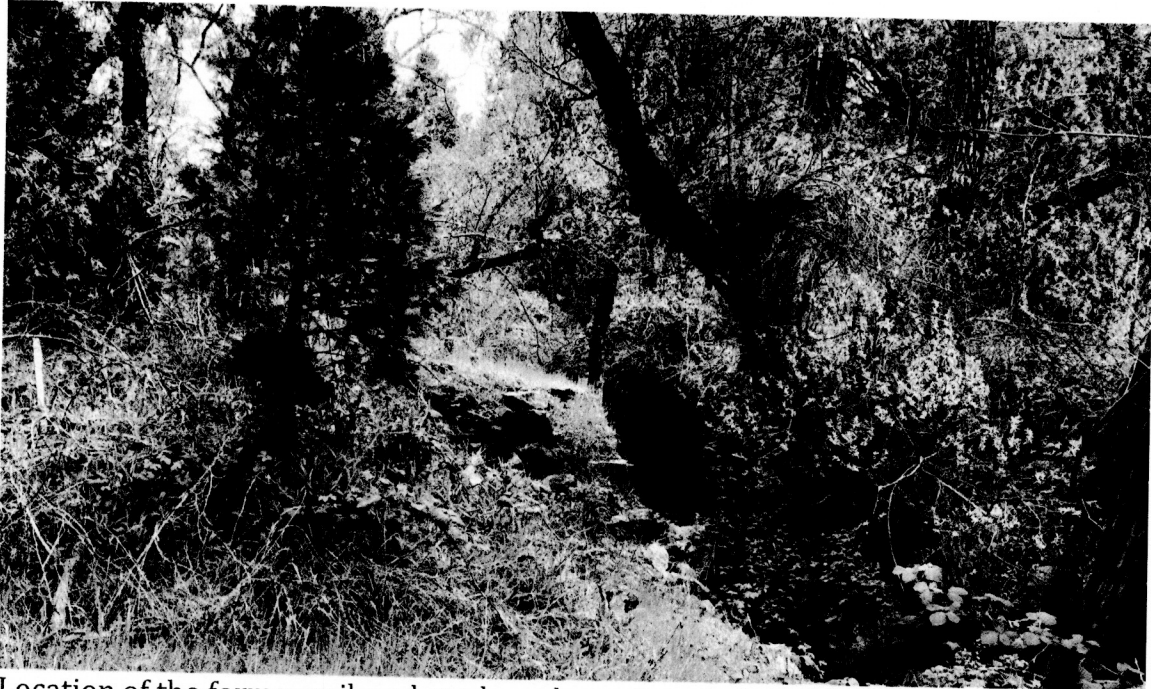
Location of the former railroad grade and granite trestle abutments viewed from the southwest. The simple wooden trestle used by the railroad was laid across the top of both abutments.
