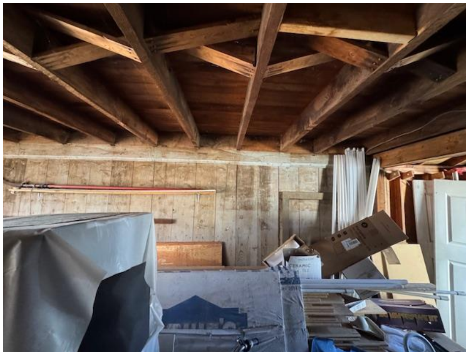
Photograph 7: View looking inside the barn towards the west wall and showing rebuilt ceiling framing for the upper floor.
