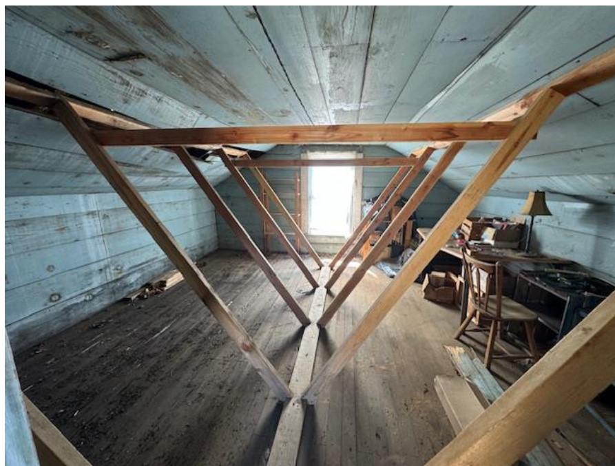
Photograph 8: View south at the upper attic area with bracing used to secure the ceiling from collapse.
