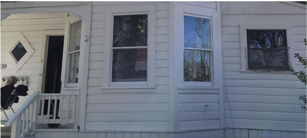
Image of replaced windows from applicant (lower level windows)
